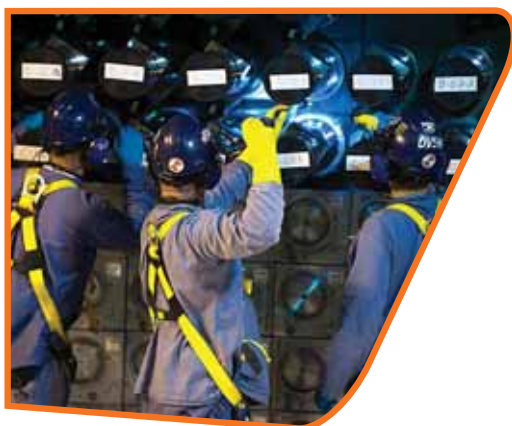
Workers install one of the 380 fuel channels in the calandria vessel at the Point Lepreau Generating Station.
