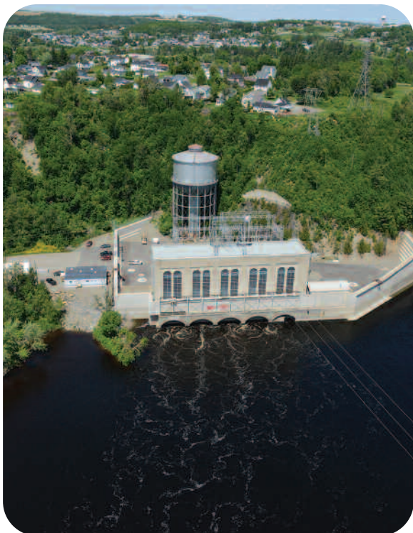
Grand Falls Generating Station
