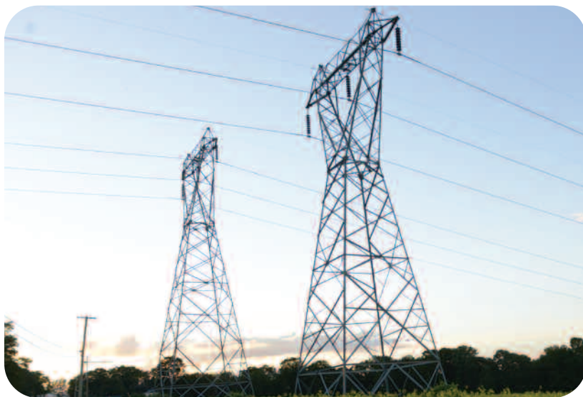
345 kV transmission towers in Keswick, NB
