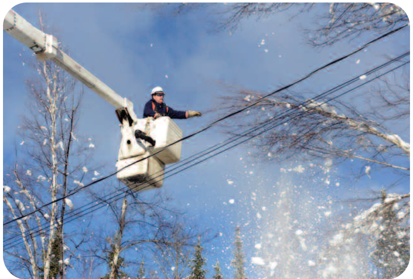
Myles McCurdy, power line technician, removing tree limbs from distribution lines, during a winter storm.
