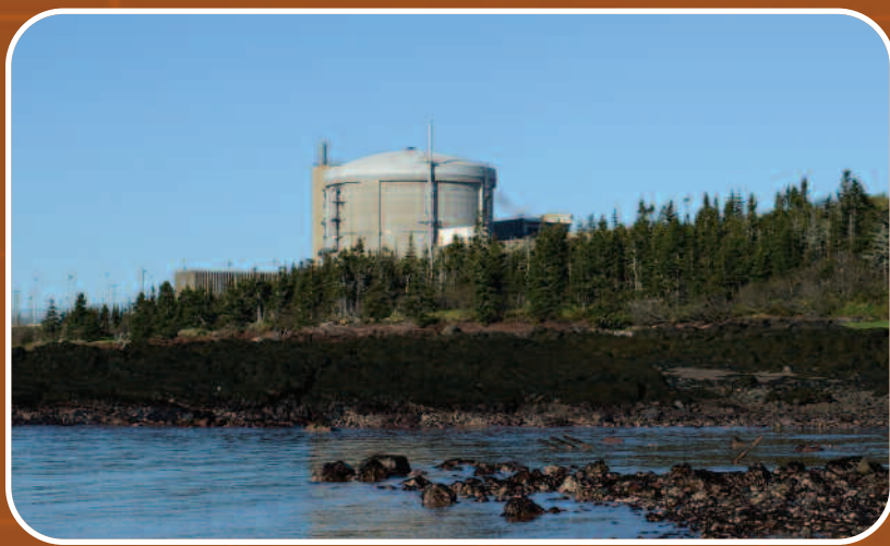
Point Lepreau Generating Station
