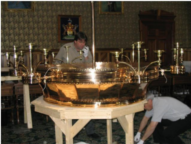
*Middle left: Keith Campbell of Acu-Bright (centre) and Steve Plante reassemble the frame of the south chandelier indicating the detail of work required to rehabilitate the bent frame.*
